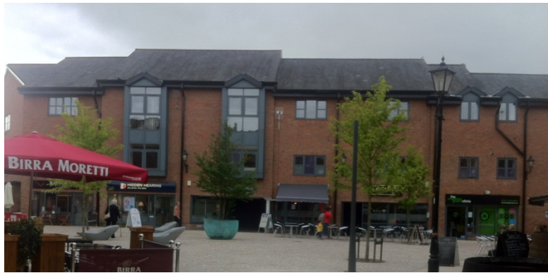
Modern shop fronts on the south side of Goose Green
