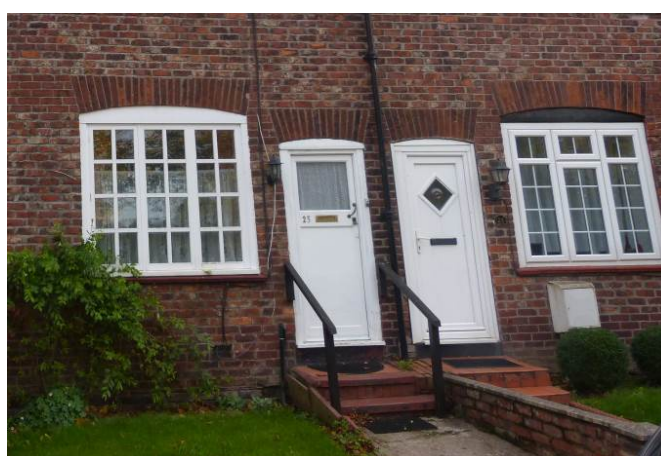
An original style window and door on the left; on the right, a modern replacement door in a similar style and thick-framed UPVC windows.
