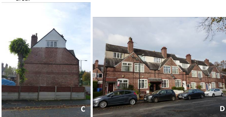
C An end elevation showing the unusual section shape of the terrace.
