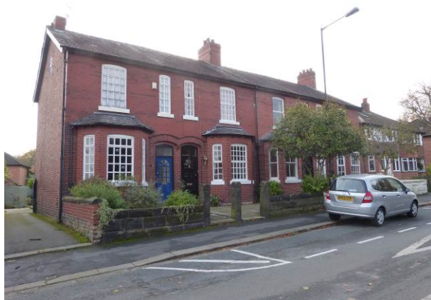
Typical examples of Style Two on Weldon Road
