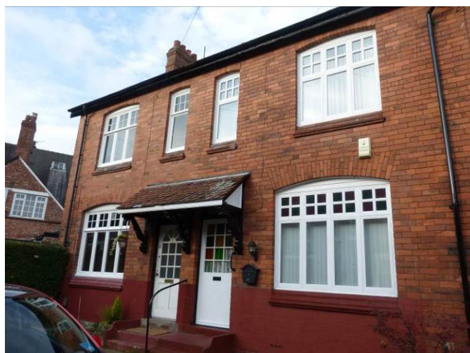
A typical example on Weldon Road
