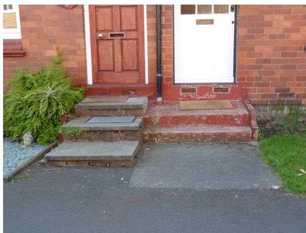
Possible original steps to the right on Pollen Road, with replacement steps on the left
