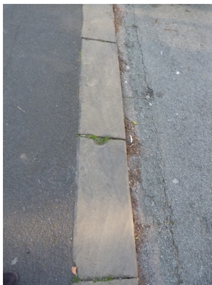
Original kerb stones on Weldon Road
