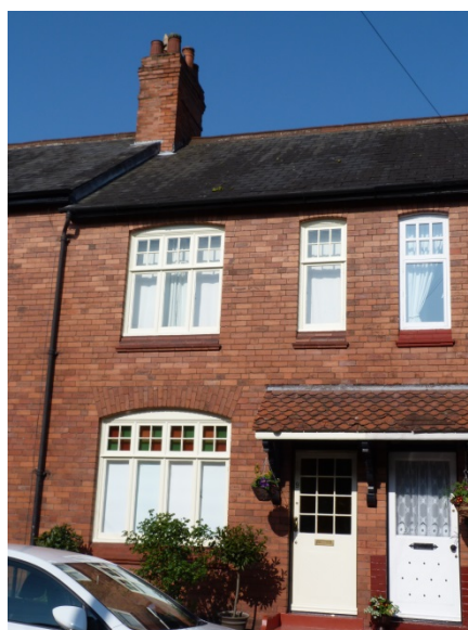
No.9 Weldon Road with surviving original windows and door
