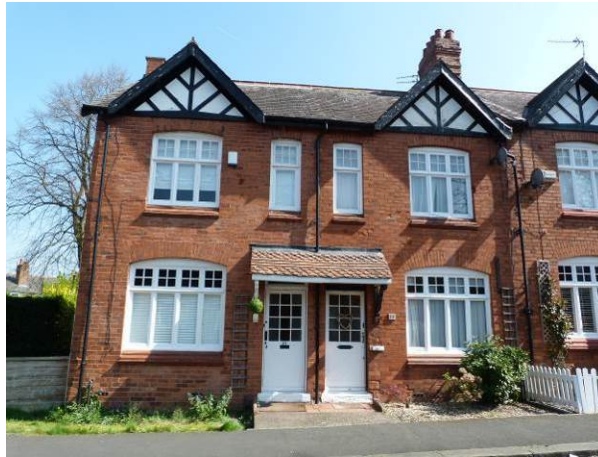
Two style six houses with surviving original windows and doors at Nos. 57 and 59 Lock Road
