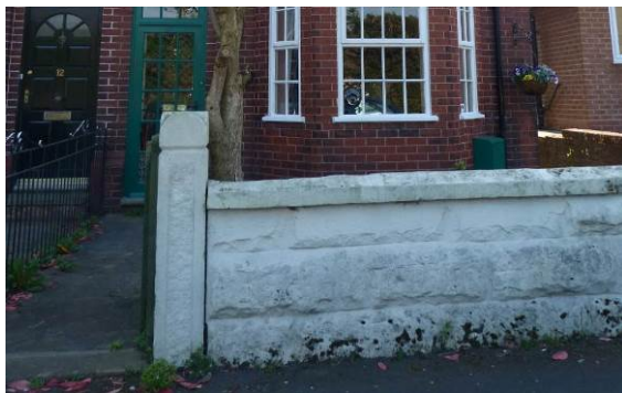
Original stone wall and gatepost at No. 10 paving Weldon Road, though this example has been painted inappropriately
