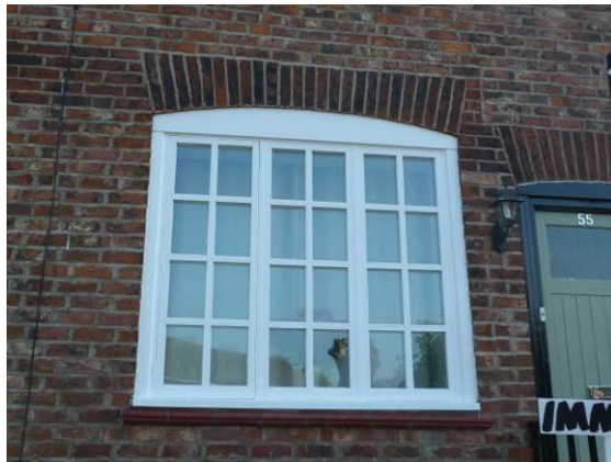
Timber framed window at No. 55 Lawrence Road
