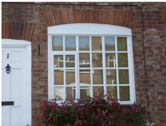
Timber framed window at No. 1 Place Road
