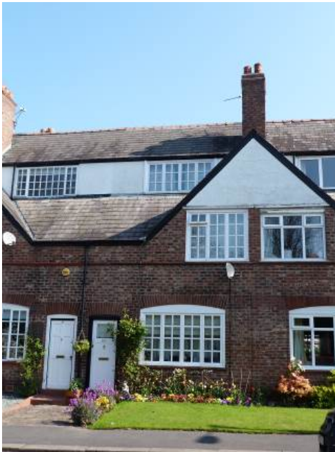
No. 89 Lawrence Road with original door and appropriate windows
