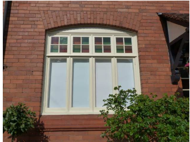
An original window at No. 9 Weldon Road
