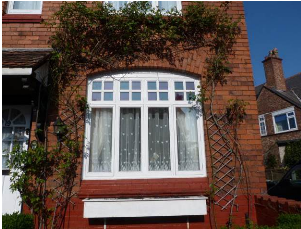
An original window at No. 19 Weldon Road
