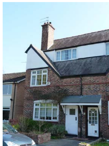
Porches added to Nos. 79 and 81 Lawrence Road
