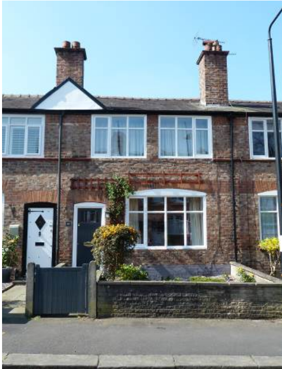
Original windows and doors at No. 69 Lock Road
