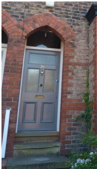
Original door at No. 26 Weldon Road
