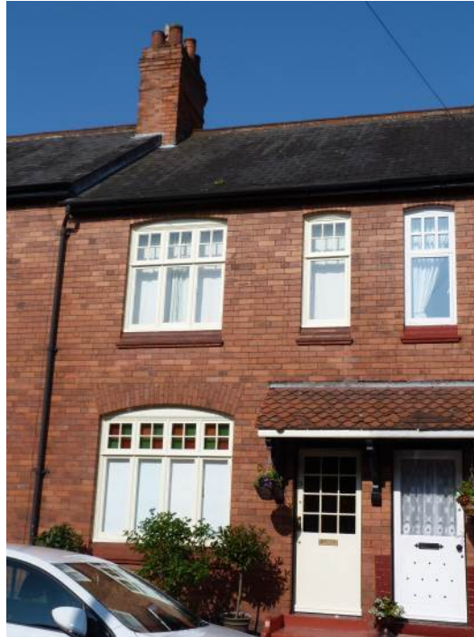
No. 9 Weldon Road, a typical style four house with original windows and doors
