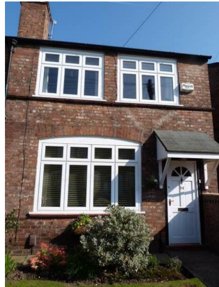
uPVC windows which are a more successful example, though with thicker frames than the original, at No. 14 Place Road
