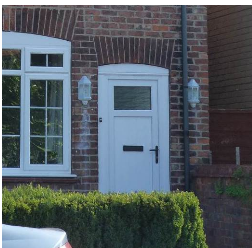
uPVC door in the original style at No. 63 Lawrence Road but with a chunkier appearance than the timber versions
