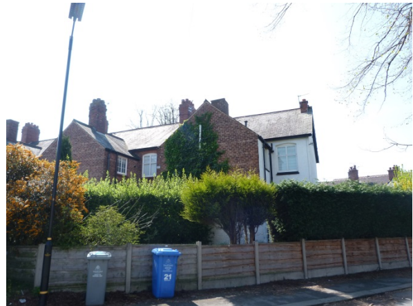
Two storey original rear projecting blocks on the back of Lock Road houses, with probable original timber windows
