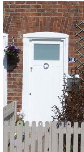
uPVC example of a door which follows the design of the original doors, No. 12 Bemrose Avenue
