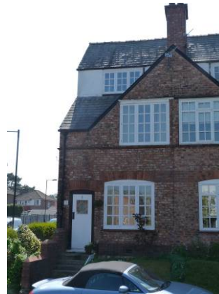
Appropriate windows at No. 1 Bemrose Avenue
