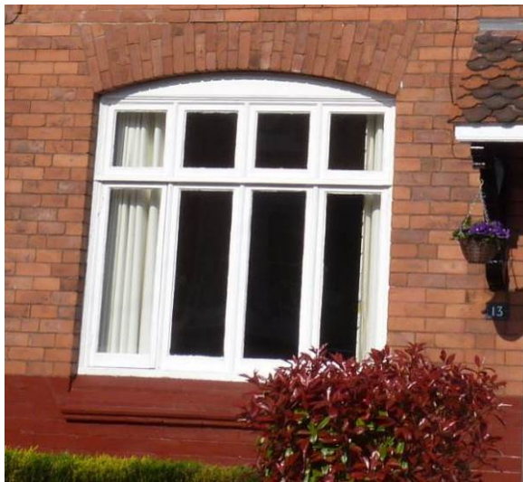
Ground floor window to No. 13 which lacks the groups of four small upper panes
