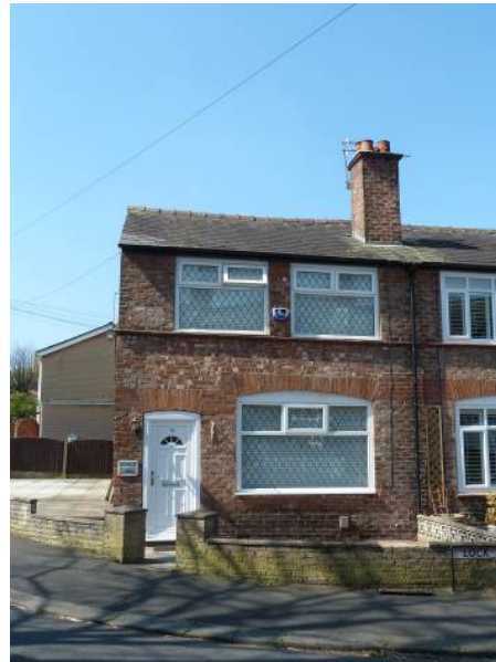
Inappropriate faux-lead windows at No. 72 Lock Road, with frames that do not match the original composition
