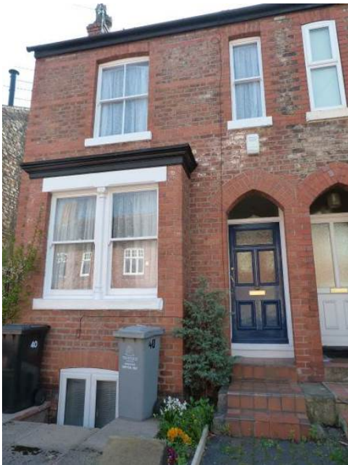
Appropriate original timber sashes at No. 40 Weldon Road. Note the column between the two ground floor windows
