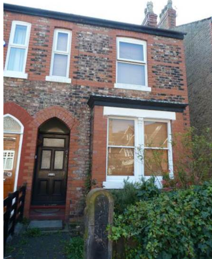
Appropriate timber sash windows on the ground floor of No. 30 Weldon Road, though the first floor windows are inappropriate uPVC replacements
