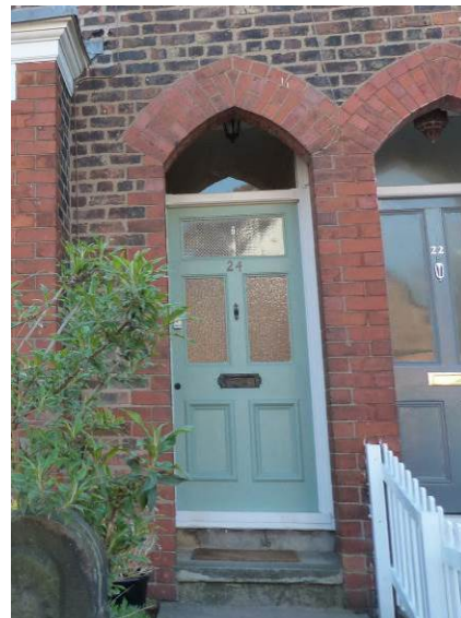
Original door at No. 24 Weldon Road
