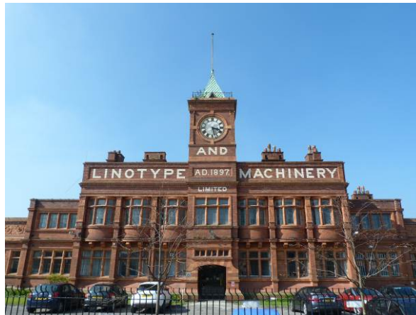
The main elevation of the Linotype Works
