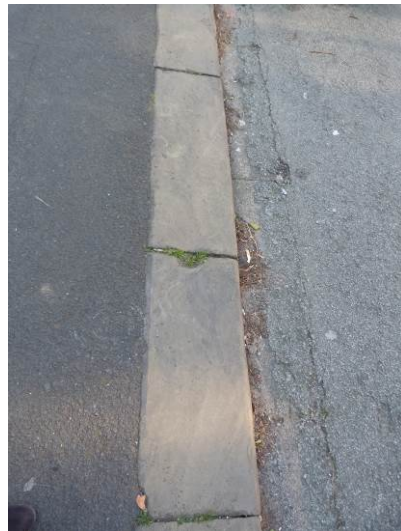
Historic kerb stones on Weldon Road
