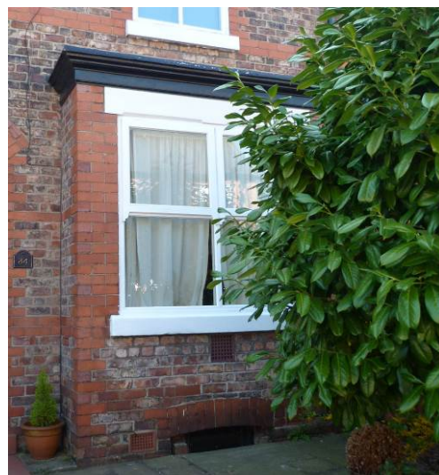
Less successful uPVC designs to No. 34 Weldon Road, which mimic sash composition but are top hung, resulting in odd proportions to the frame
