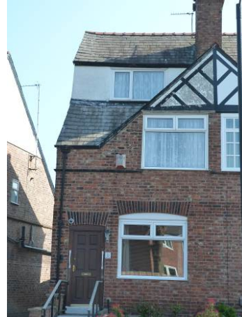
Inappropriate windows at No. 53 Lawrence Road
