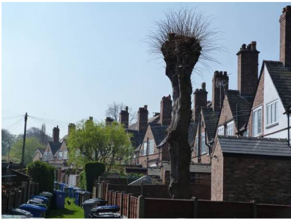
The rear elevations of Lawrence Road
