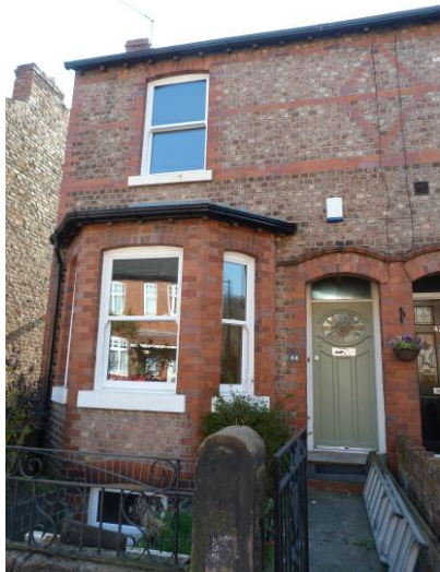
uPVC sash windows at No.44 Weldon Road
