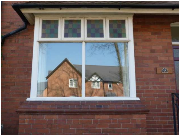
Style Seven: Original window frame to No. 15 Norman Road, though with possible replacement coloured glass panes
