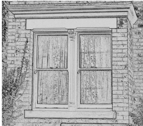
Sketch of original window, including moulded horns to the underside of the top sash
