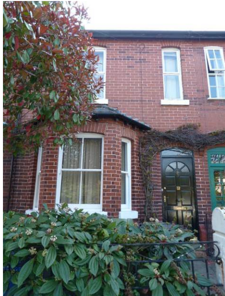
A typical style two house at No.12 Weldon Road. This example has original windows but a replacement door
