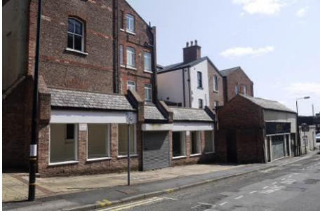
Vacant shops and heavy-duty security provision on Post Office Street
