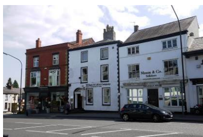
late 18 th century buildings at 8-12 Old Market Place retaining traditional features such as windows and railings but with deteriorating and painted fabric and some inappropriate window replacements
