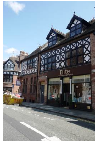
Example of an appropriate shop front
