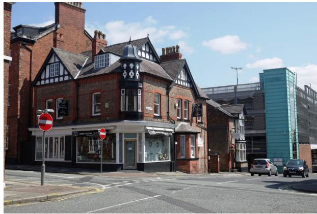
Arts and Crafts detailing on an Edwardian development on Market Street
