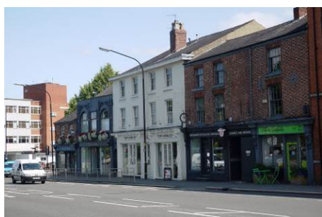
Good examples of traditional shop fronts and buildings in good condition at 30-36 Church Street
