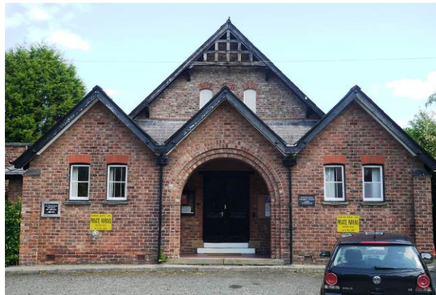
Unitarian Sunday School is also in need of maintenance
