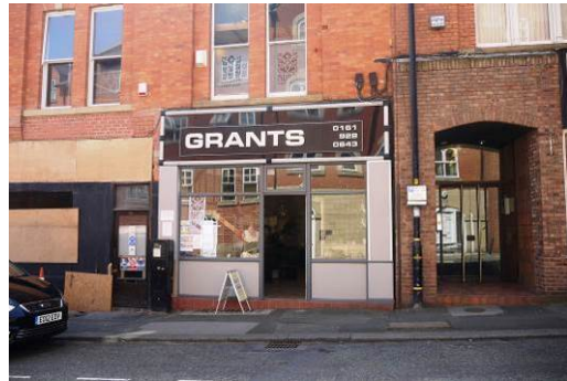
Inappropriate shop front using aluminium frames, plastic fascia and reflective glass
