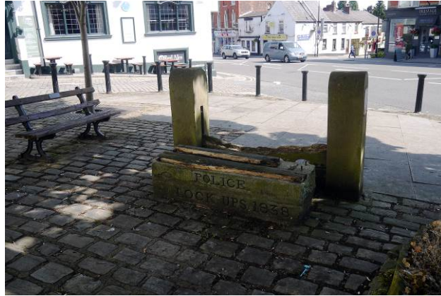
Replica stocks on the Market Place, currently in a poor condition
