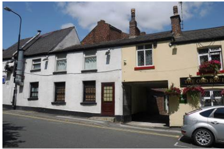
Replacement windows and doors are detrimental to these late 18 th century properties, particularly the faux-leaded lights
