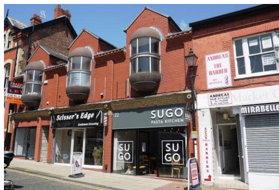
Late 20 th century shop units are interesting examples with upper floor display windows that should be retained
