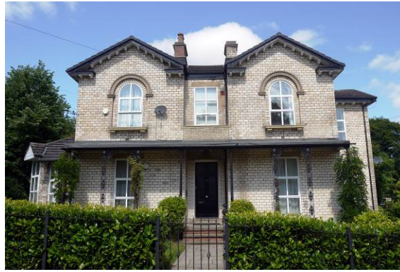
Example of the typical architectural features of the area including deep eaves and brackets and wide buff bricks. Windows have been replaced with inappropriate uPVC windows and an unsightly extension has been added (left of image)
