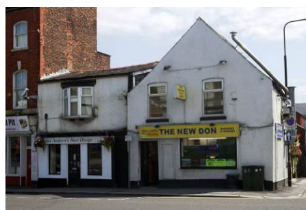
Shops on the Old Market Place in a poor condition, with inappropriate signage, modern windows and painted brickwork.
