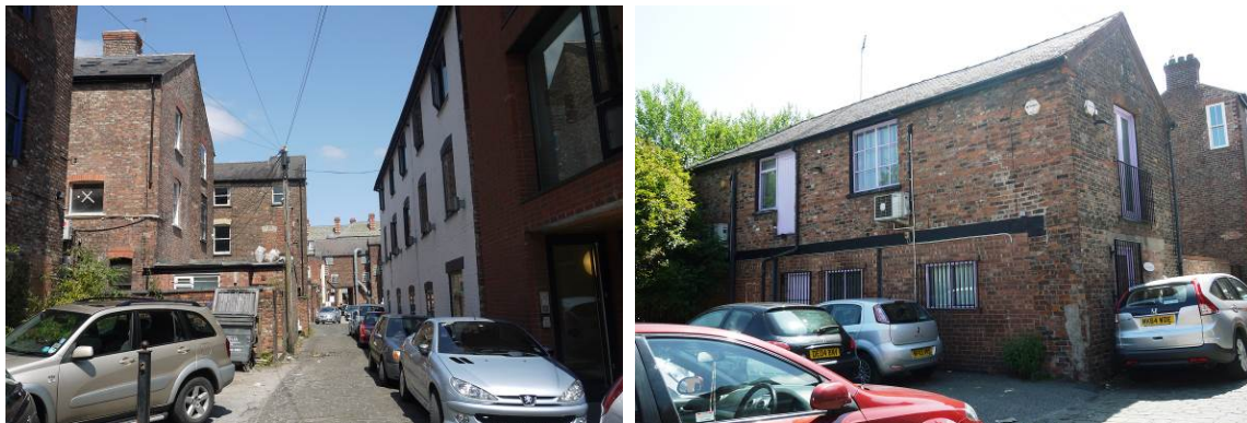
Industrial (now renovated) buildings along Back Grafton Street
