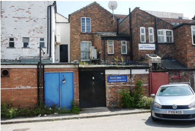
Rear of Stamford New Road, within Lloyds Square, showing intrusive air conditioning units and some painted rear elevations.
