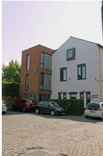
New development associated with former industrial buildings on Back Grafton Street
