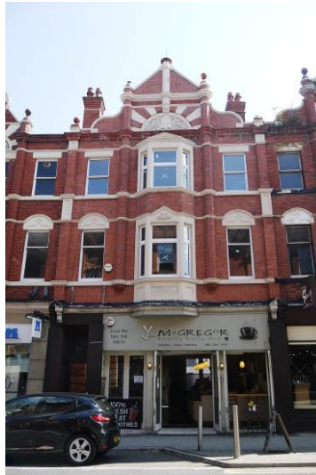
Good example of a well-maintained property (31 Stamford New Road). However the stone work has been inappropriately painted
