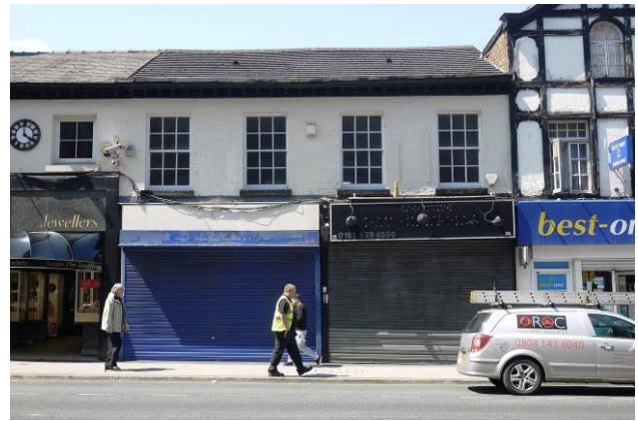
24-30 Railway Street are three properties that have been extensively altered and have potential for enhancement. Note the inappropriate (and vacant) shop fronts with roller shutters and recently painted façade. Traditional windows survive on 24-26 but have been replaced with uPVC in an inappropriate square design at 30.
