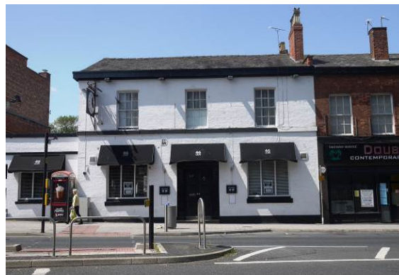
The painted façade and replacement door and ground floor windows of 46 Railway Street (formerly The Downs Hotel). The simple design of these buildings leaves them vulnerable to harmful cumulative change over time.
