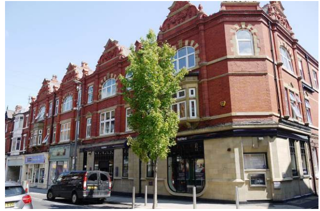
17-23 Stamford New Road, a commercial parade in good condition with a limited amount of vacancy
