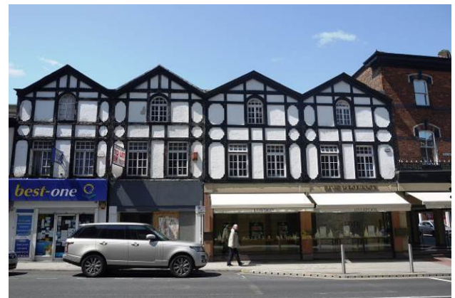
Example of Cheshire Vernacular at 16-22 Railway Street
