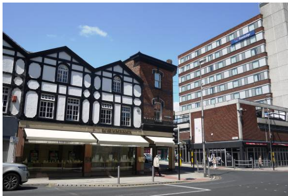
Appropriate use of canopies within the Conservation Area
