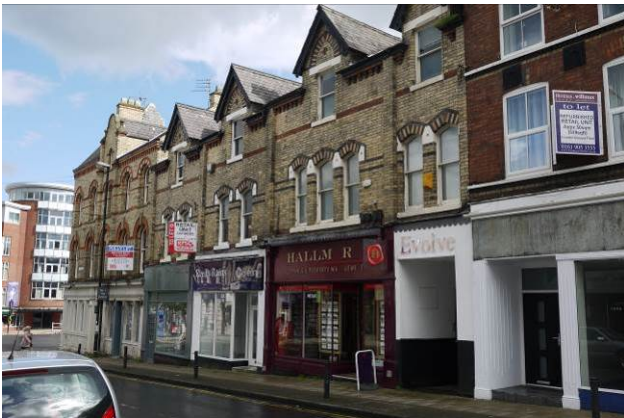
Late Victorian buildings in commercial and retail use on the lower Downs with some poor ground floor frontage alterations
