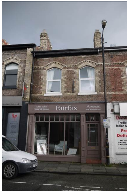
Traditional replacement shop front on Oxford Street
