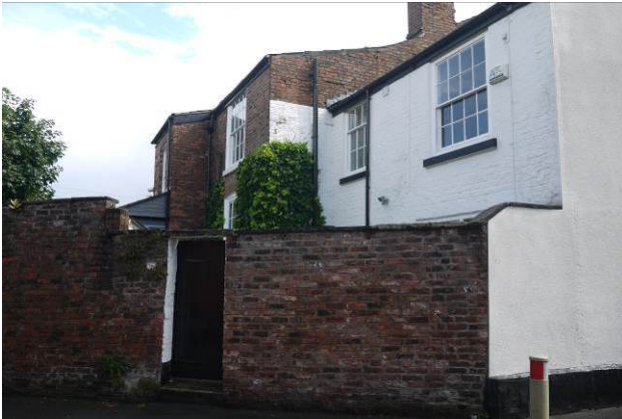
Rear elevations to properties along The Downs viewed from New Street
