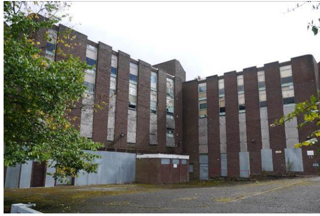
The derelict YWCA building on St Johns Road
