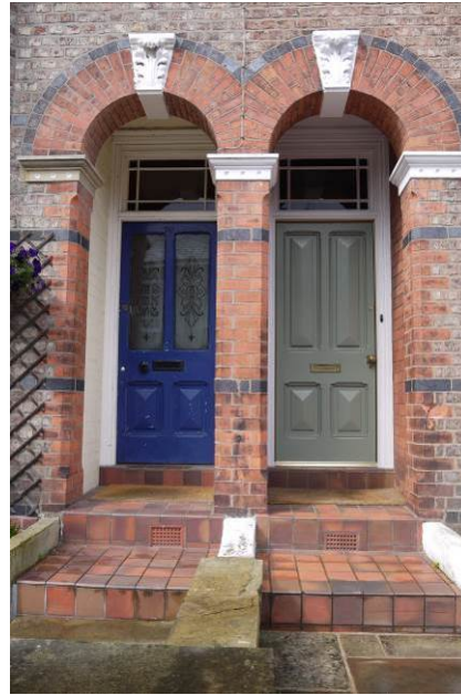
Original doors on New Street
