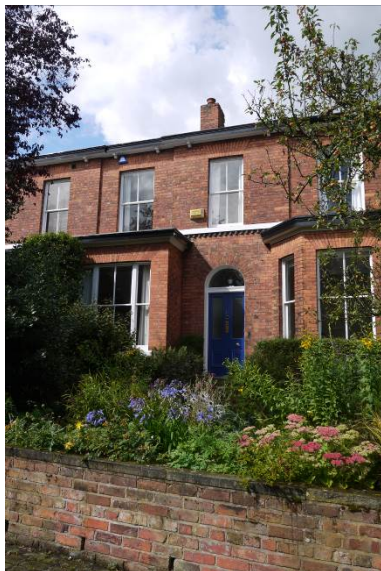
Mature raised gardens behind low brick retaining walls are common
