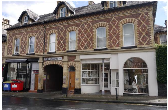
Shop fronts along the lower Downs
