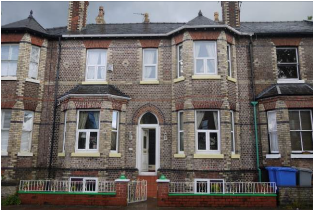
Substantial Victorian terraces, many have suffered from inappropriate replacement of features such as windows, doors and boundary walls
