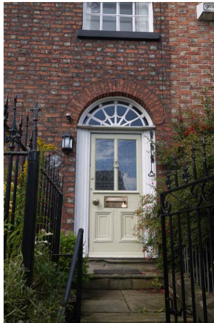
Original fanlight, bell pull and railings on No. 42 The Downs. The door is a slightly later replacement with stained glass
