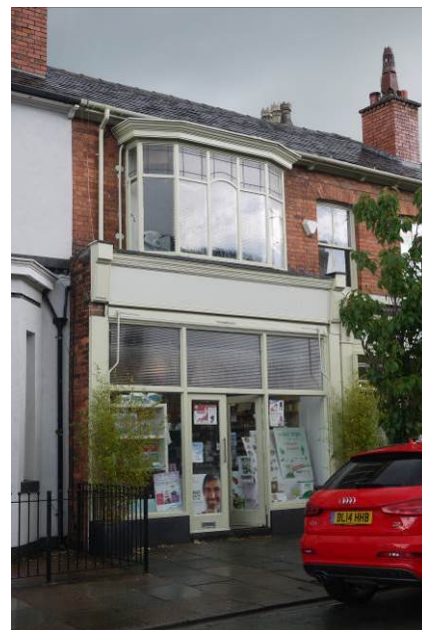
Local details include eye catching timber bow windows and shop fronts along Oxford Road
