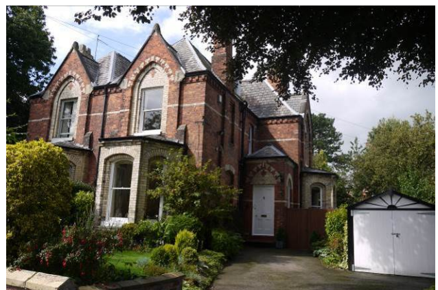
High Victorian architecture making use of polychromatic brickwork and fanciful Gothic gables and arches
