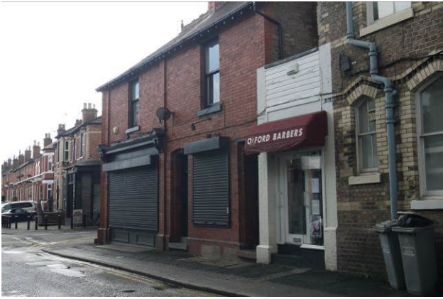
Inappropriate use of solid security shutters on Oxford Road
