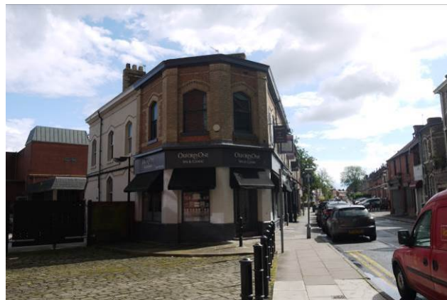
An appropriate use of awnings within the Conservation Area, no. 1 Oxford Road
