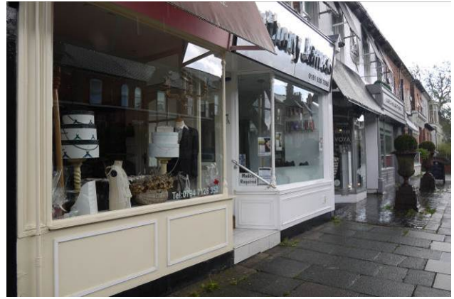
Original shop fronts with stall risers, slender glazing bars and panelling. The fascias are not appropriate
