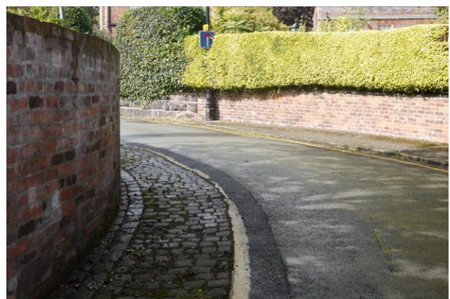
Traditional stone setts and more modern surfaces sit side by side on Lyme Grove
