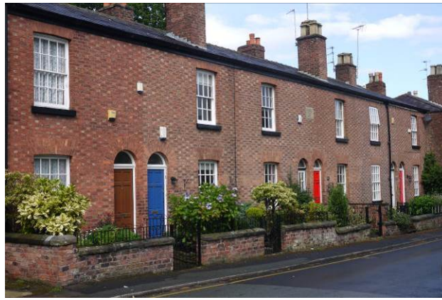
Simple classical terraced houses with round arched doors, 8 over 8 sash windows and Flemish bond brickwork at 46 New Street
