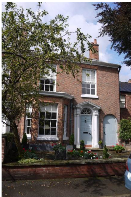
Details such as bay windows, 6 over 6 windows, broken-pedimented porch and rubbed brick arches
