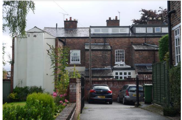
Rear elevation showing rendered outriggers, ground floor extensions and converted attic spaces with additional windows
