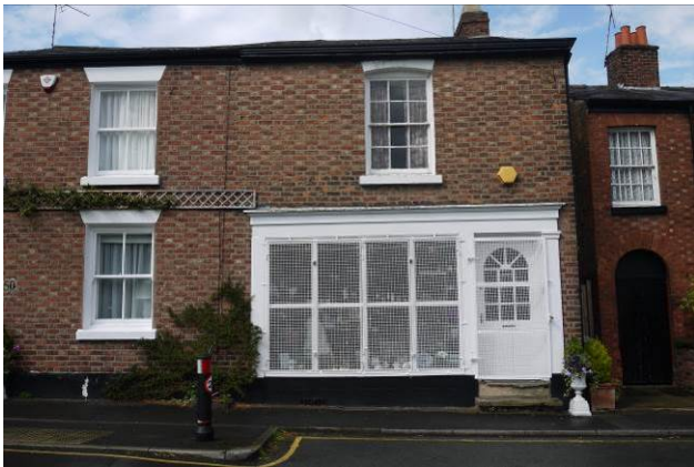
An original shop front within Character Zone A on New Street
