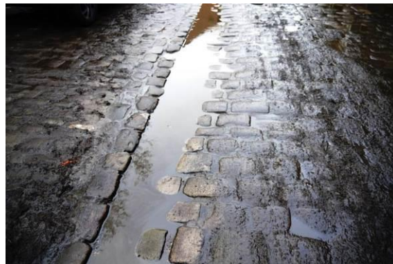
Paving at the north end of Church Lane
