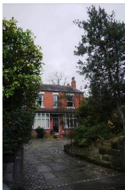
Villa at the northernmost end of the character zone on the west side of Church Lane
