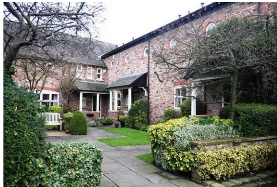
View of the northern range of the Mill development
