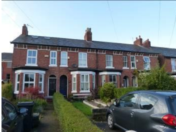
The unusual timber eaves cornice extant on Nos. 2 to 5 only
