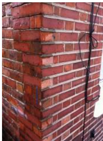
Hard cementitious ribbon pointing to front elevation
