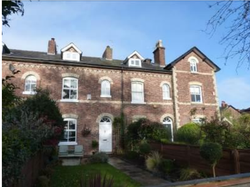
The south-east end of Brogden Terrace, showing the dormer gables, mismatched chimney pots, varying window styles and contrasting yellow brick detailing
