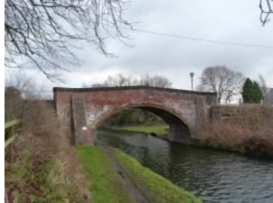
Dunham School Bridge
