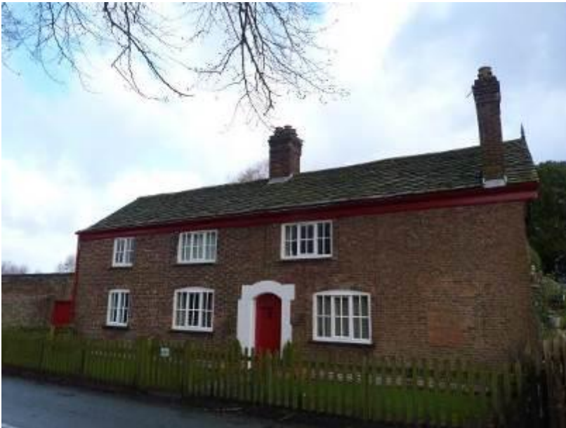
101 Woodhouse Lane - street elevation
