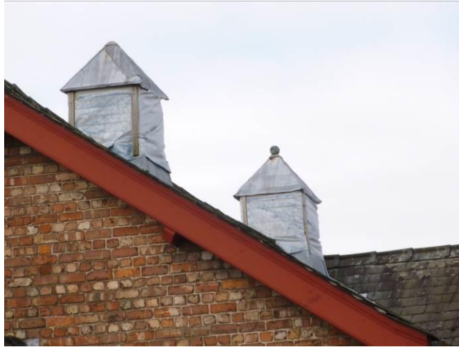
Sheeted ventilators to Village Farm out-buildings
