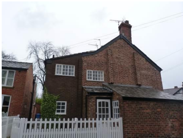
End elevation of Rose Cottage
