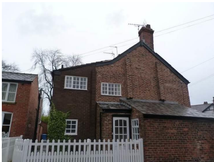
End elevation of Rose Cottage
