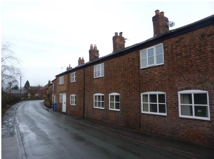
Terraced cottages on Woodhouse Lane
