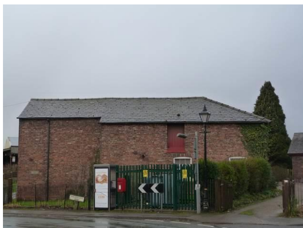
Substation in the centre of the village
