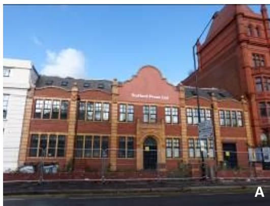
A. The Chester Road elevation of the Trafford Press Building.
