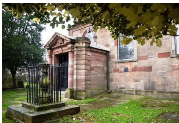
The south elevation of the church, showing the 1909 porch and the listed sundial
