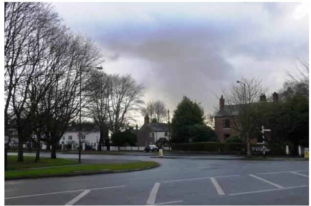
View east into the Conservation Area from the B5158
