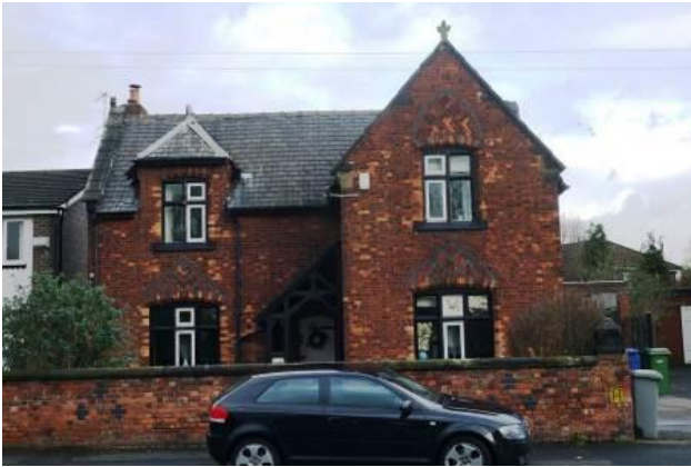
350 Church Road, the former school house
