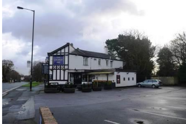
The large car park to the rear of the Church Inn.
