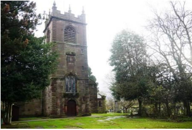
West elevation of the church
