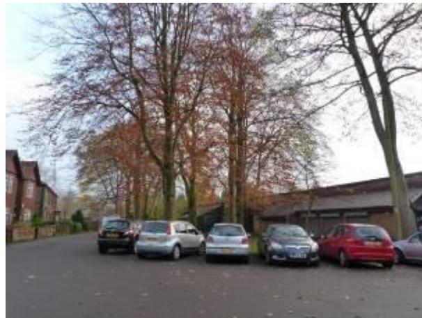
20 th -Century lean-to sheds against the north side of the Walled Garden
