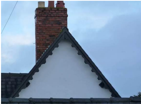
Detail of later applied barge boarding
