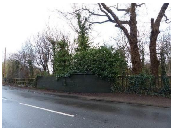
Original bridge over the River Mersey
