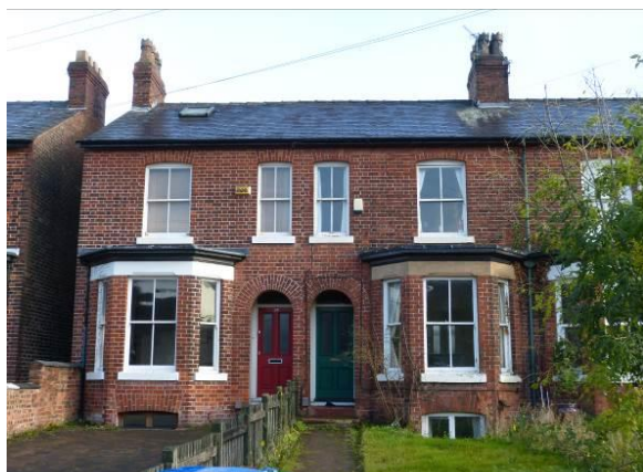
A typical pair of Brogden Grove houses, both with early replacement windows (discernible for their slimmer frames but straight top edge). The doors have been replaced in an appropriate style (see paragraph 2.3.5).
