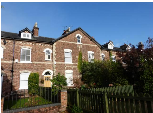
The central block of Brogden Terrace, with attic dormers on either side and detailing picked out in contrasting stock brick.
