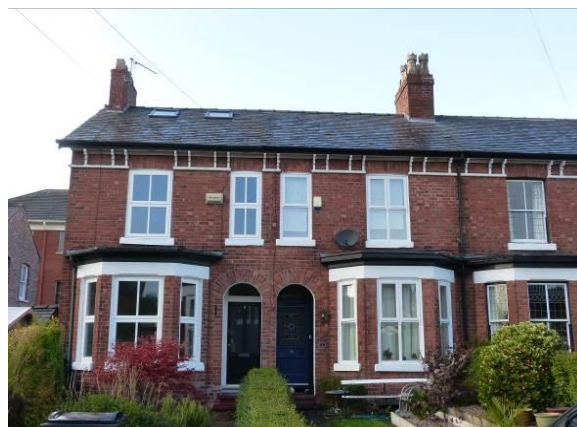
The eaves cornice on Nos. 2 to 5 Brogden Grove.
