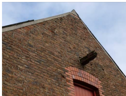
Different bricks on one of the agricultural buildings
