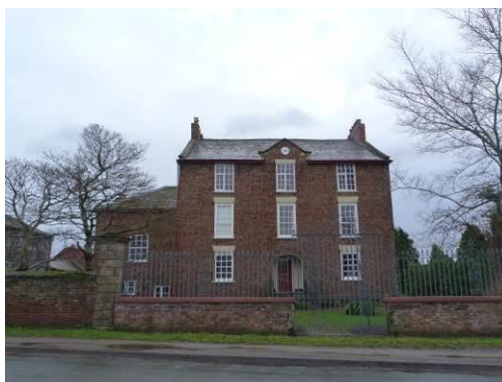
Manor House Farm (the former Dower House), with its prominent tall railings, gates and rusticated end pier indicating its historic status
