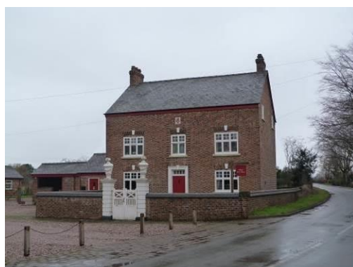
Village Farm House, with its prominent gateposts and forecourt wall, and temporary stanchion and chains
