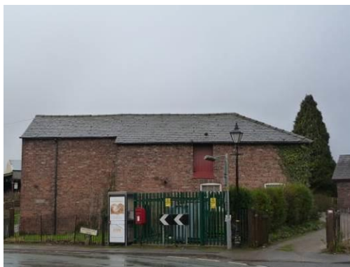
The incongruous sub-station and phone box
