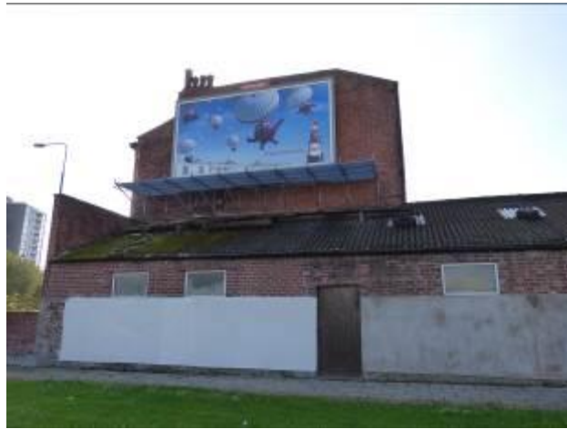
Inappropriate modern hoarding on the side of a historic terrace
