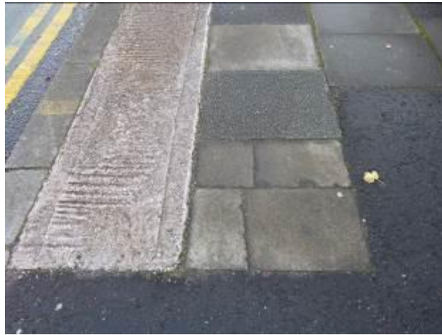
Ad hoc pavement repairs on Chester Road
