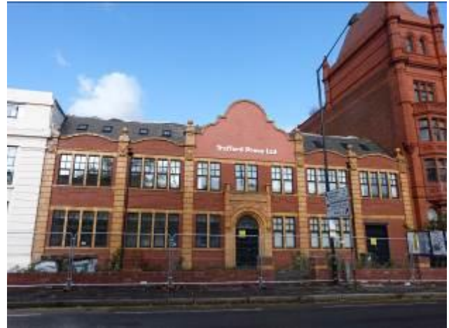
The partially-refurbished but vacant Trafford Press building
