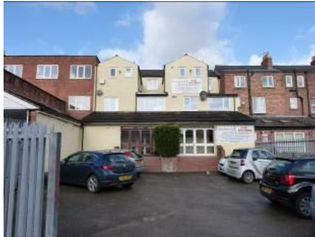
Substantial rear extension to the terraces at the south end of Chester Road
