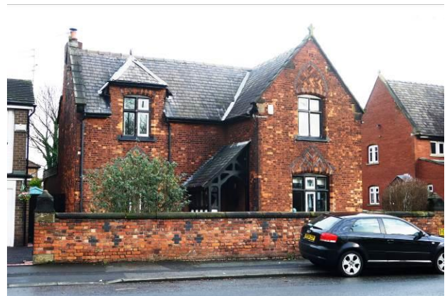
Former school house at no. 350 Church Road; note the historic boundary wall, now in a poor condition
