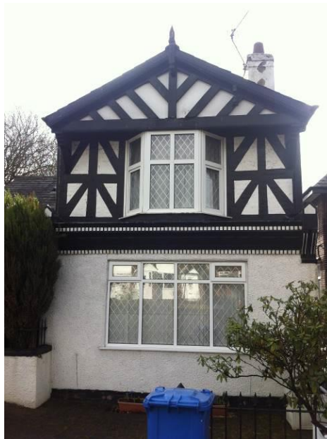
Inappropriate uPVC windows and faux leaded glazing at no. 28 The Village
