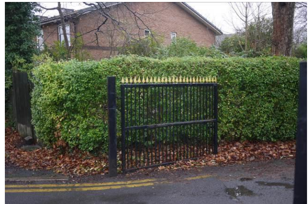
Inappropriate gates at the entrance to the park and stadium
