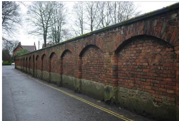
Rear wall of the walled garden area
