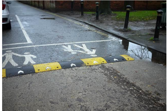
Intrusive speed bumps
