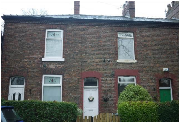
Examples of the appropriate timber and intrusive uPVC doors Longford Cottages
