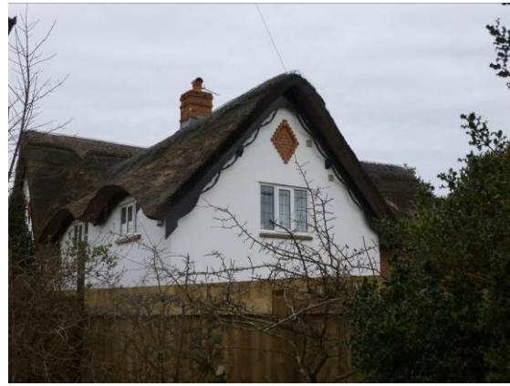
Replacement uPVC windows at 1 Wigsey Lane
