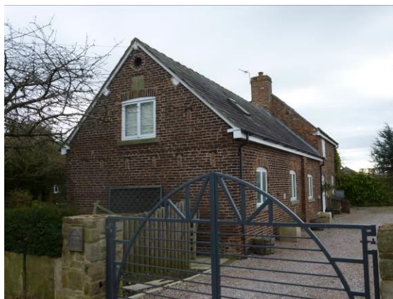
Sensitively-designed modern gates at Wigsey Cruck
