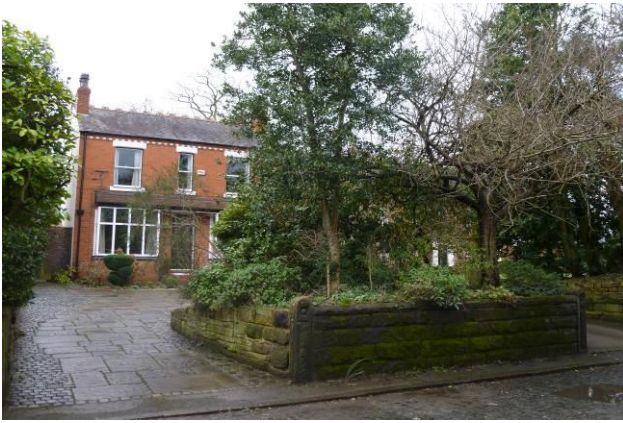
Original boundary treatment of low stone walls and gate piers
