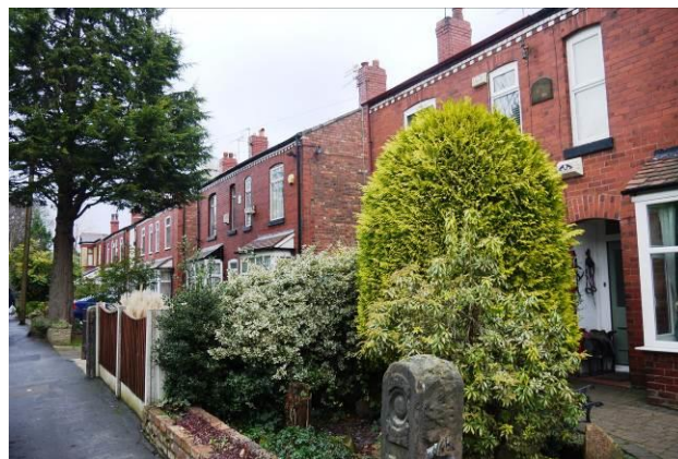
View along the east side of Church Lane
