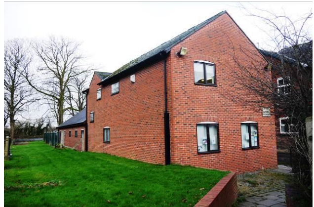
The boundary between the churchyard and the community hall
