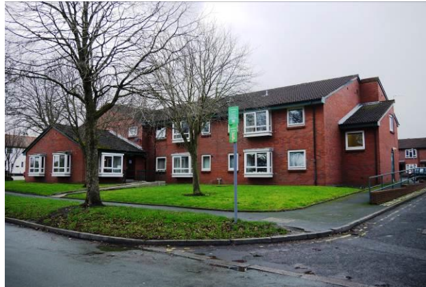
Inappropriate modern development within the setting of the Conservation Area
