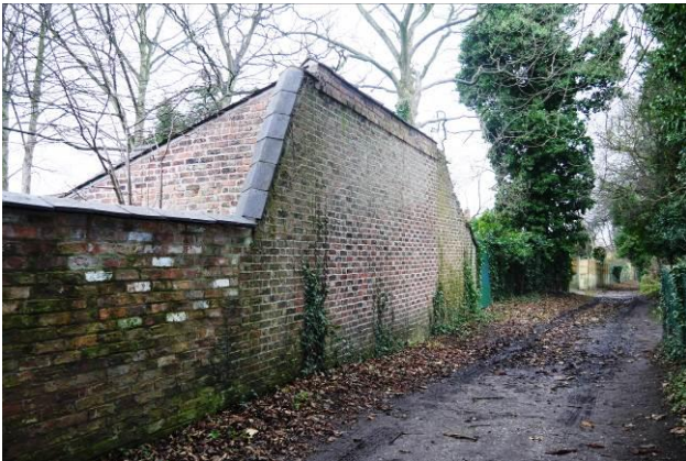
Rear boundary to Ashton New Hall
