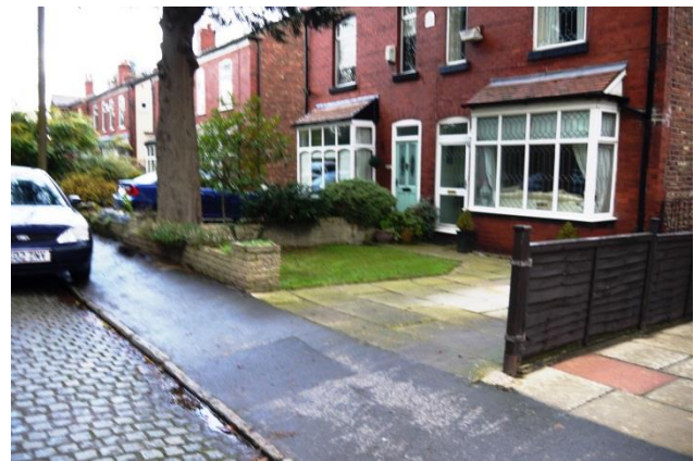
Inappropriate modern materials including concrete slabs and modern stonework. The loss of planting is also detrimental to character
