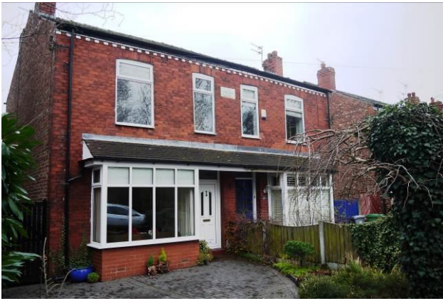
Modern setts within the driveway of Larch Villas (east side)
