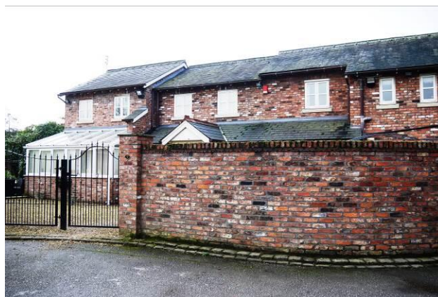
Rear of the Old Mill development showing conservatory extensions
