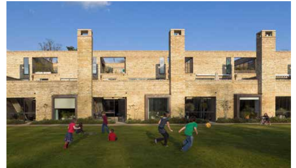
Figure 40. Reflect a Distinctive Character: respond to the historic and contemporary character of its place. For example use of local and robust materials for external elevations.
