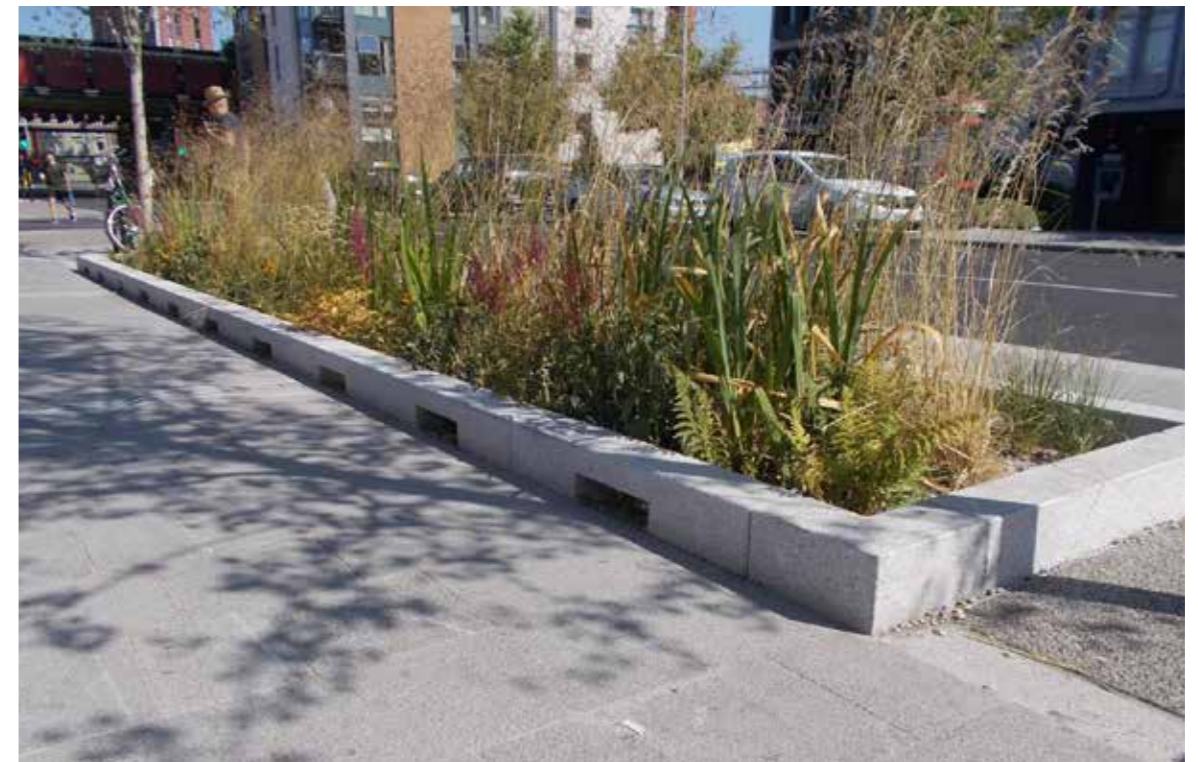
Figure 35. SUDs - Planting bed and drainage channels adjacent to a cycle lane in Salford
