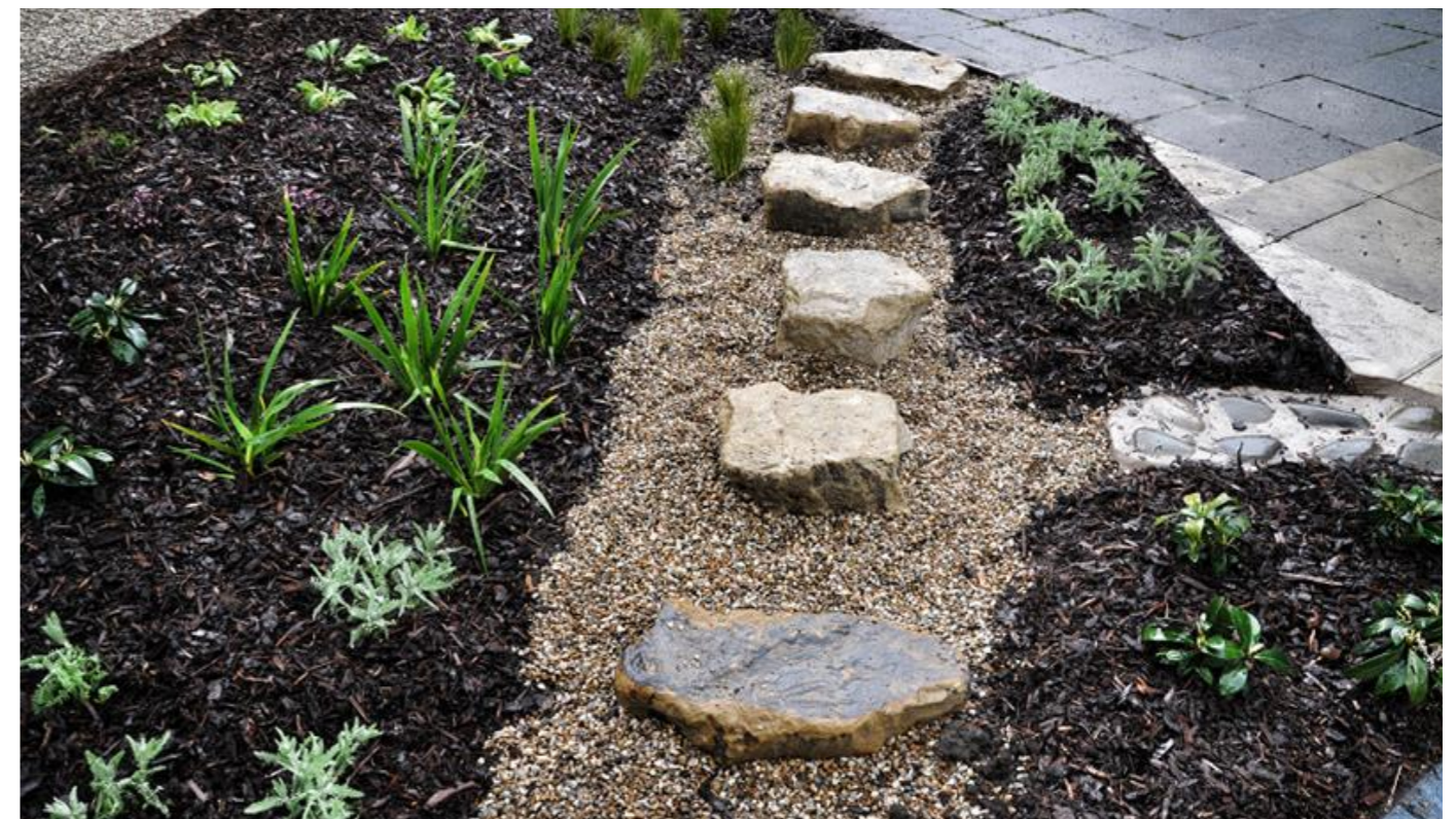
Figure 36. SUDs - Planting bed and permeable paving at Moorland Junior School, Sale Image from: https://www.susdrain.org/case-studies/pdfs/suds_awards/025_18_04_30_susdrain_suds_awards_moorlands_junior_school_suds_sale.pdf
