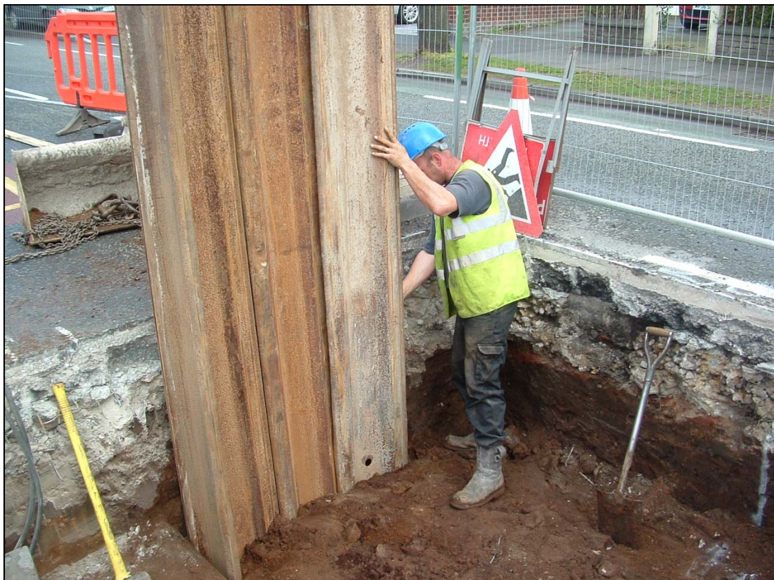
Photo 1 – Driving & stabilising the trench piles
