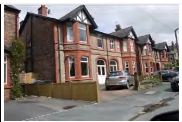
Photograph 26: Properties along Appleton Road
