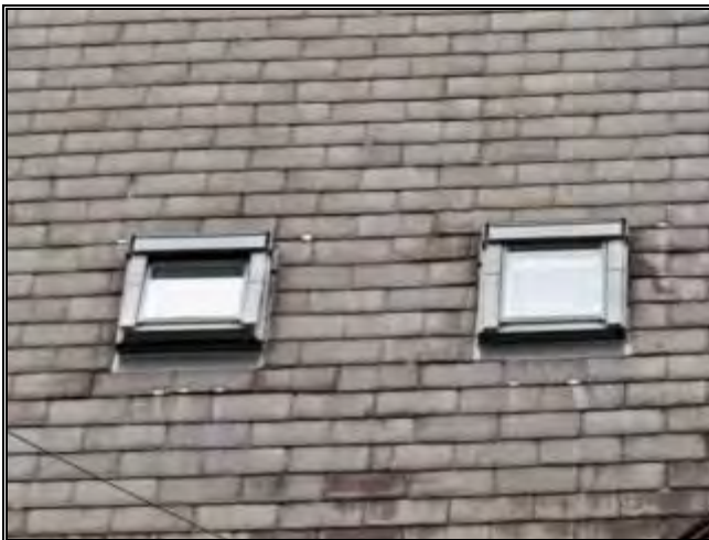
Photograph 109: Skylights on front Elevation of 3 Warwick Road
