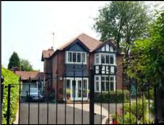
Photograph 111: UPVC Windows and door surround to 8 Harrop Road
