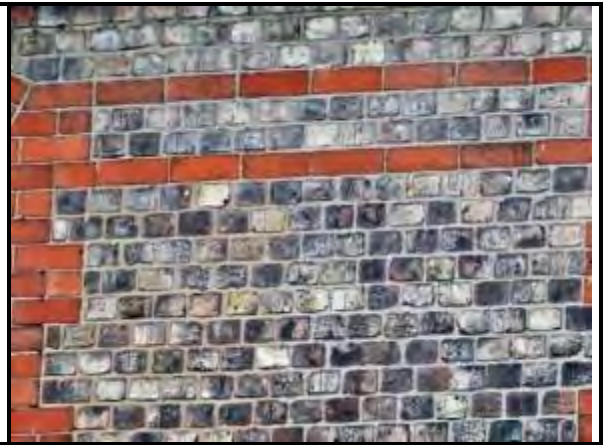
Photograph 5: Cheshire Brick with Red Brick used for Decoration
