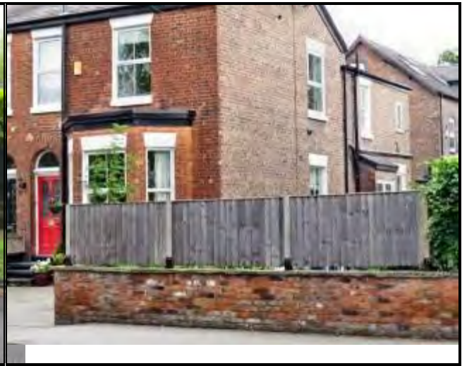
Photograph 120: Brick Wall and Timber Fencing, Ashley Road
