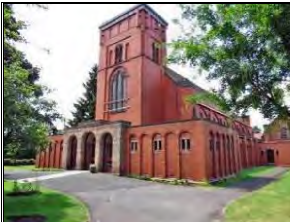
Photograph 38: Open Space around Trinity Hale Church
