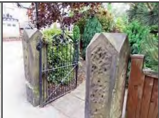
Photograph 34: Original Gate and Stone Gateposts, 1 Park Road
