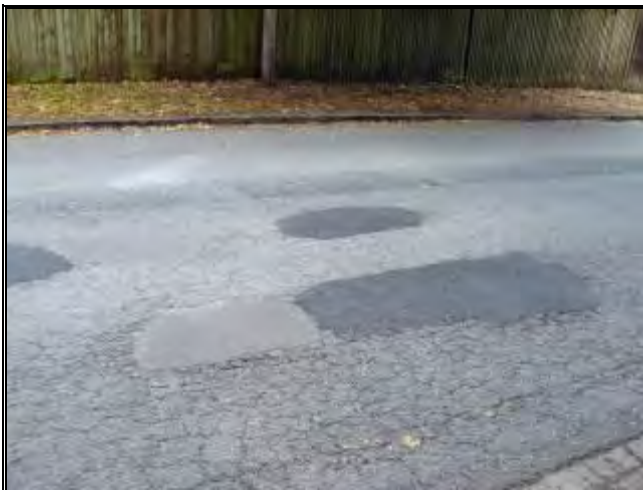
Photograph 127: Patch Repairs on Rappax Road
