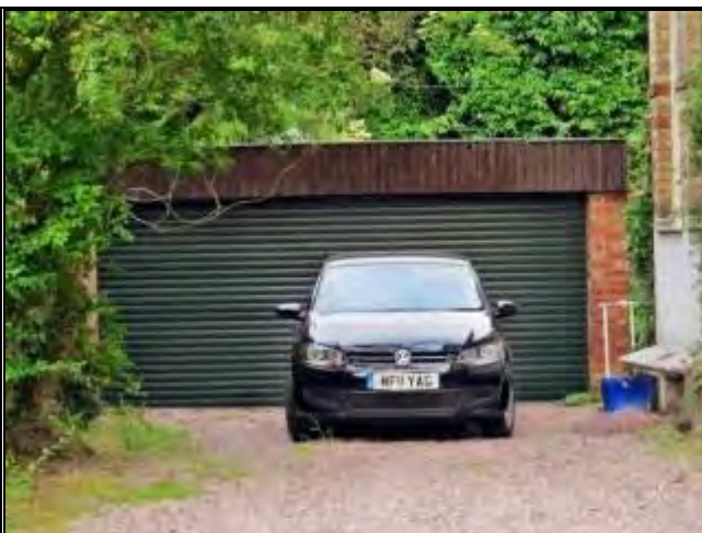
Photograph 115: Inappropriate Garage to 255 Ashley Road
