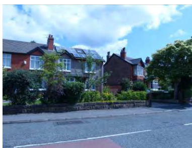
Solar panels on Arthog Road
