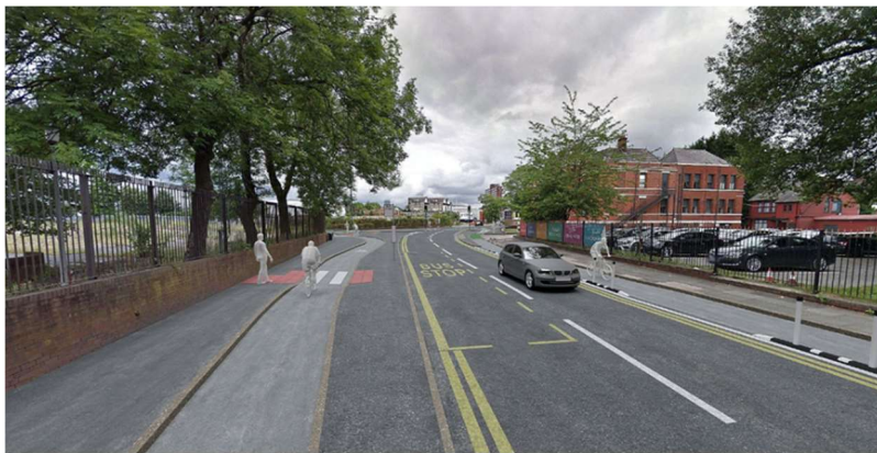
Figure 2: Talbot Road looking Eastbound.
