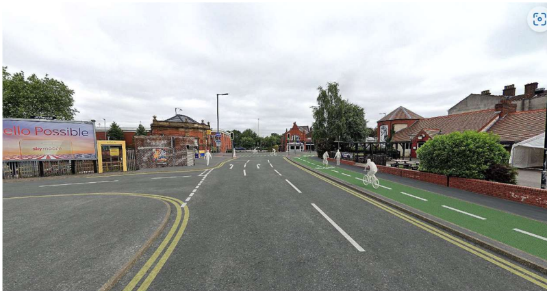
Figure 4: Seymour Grove looking northbound towards Talbot Road junction.
