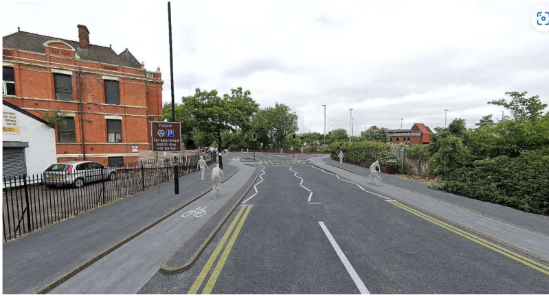
Figure 3: Talbot Road looking Westbound.
